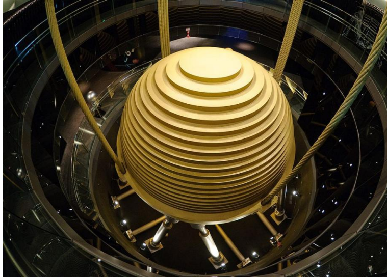
Figure 34: 660 tonne tuned mass damper system in 101 storey Taipei skyscraper [53]
